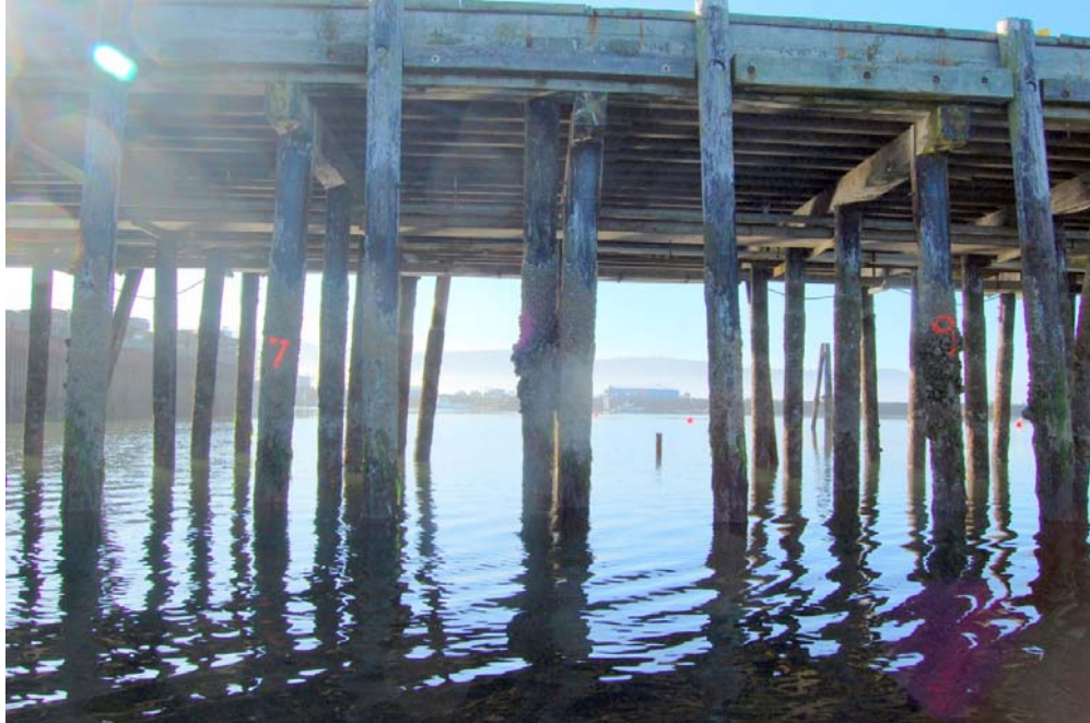
Approach Trestle Bents 7 to 9 (Photo #309) No damage noted
