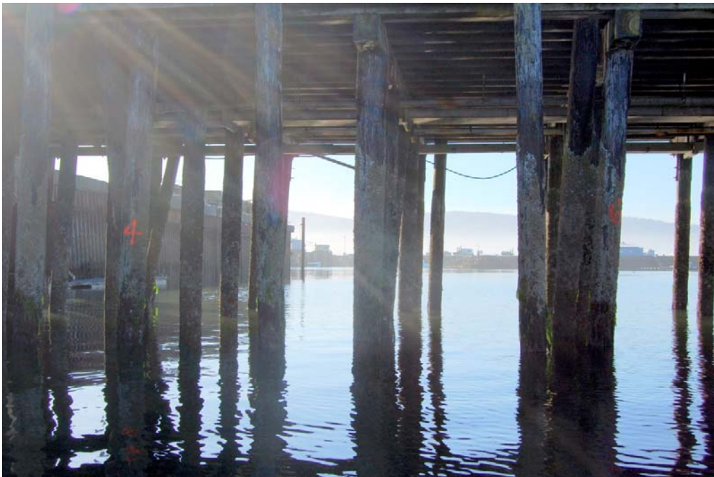
Approach Trestle Bents 4 to 6 (Photo #306) No damage noted
