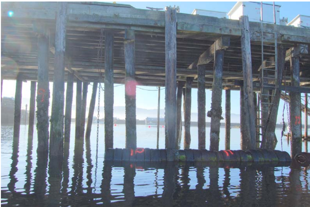
Approach Trestle Bents 9 to 12 (Photo #310) Bent steel ladder
