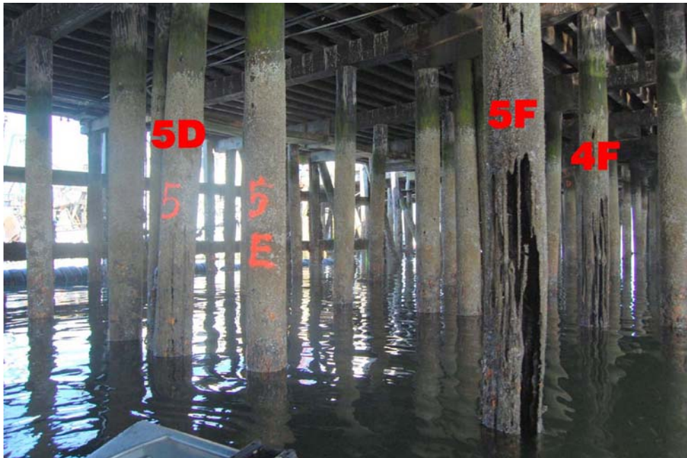
Piles 5D, 5F, and 4F (Photo #357)
