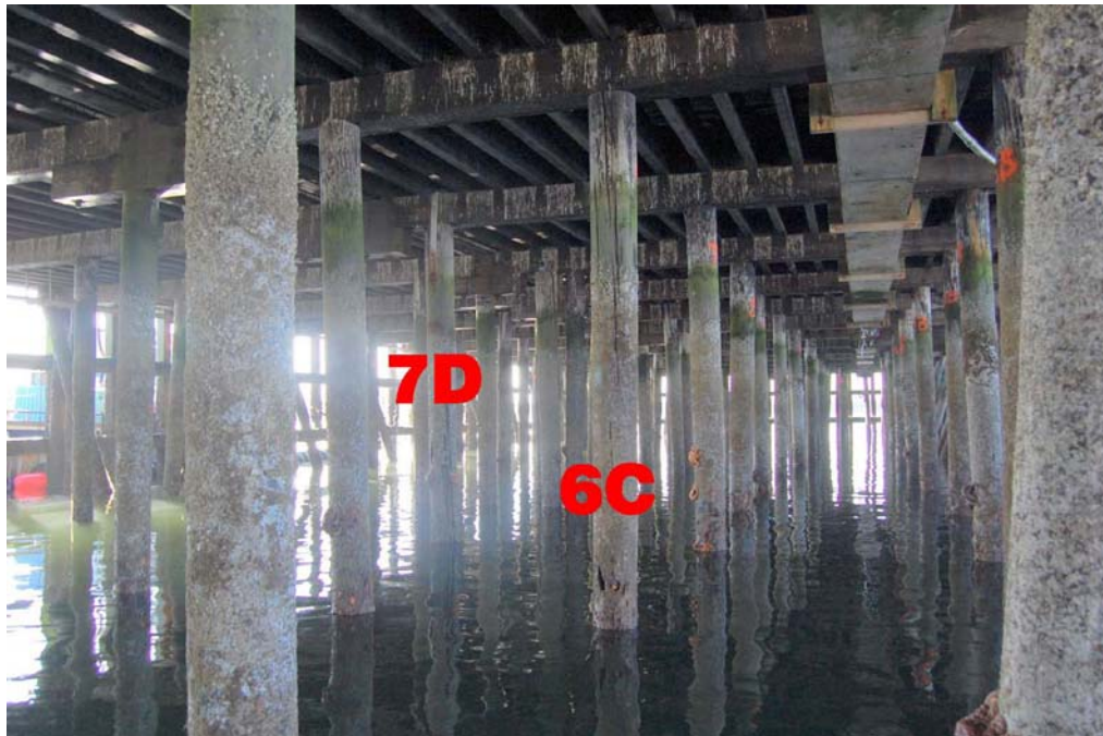
Pile 6C (Pile 7D beyond)
