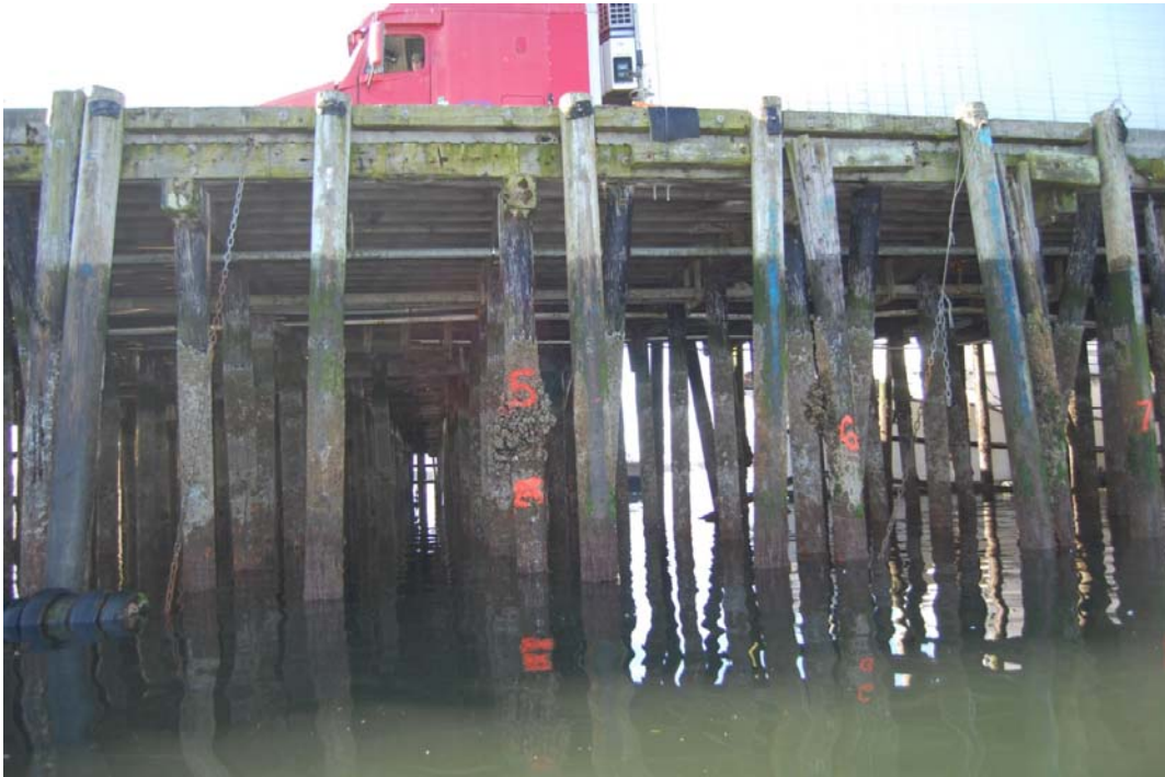
West Wharf Bents 4 to 7 (Photo #322) No damage noted
