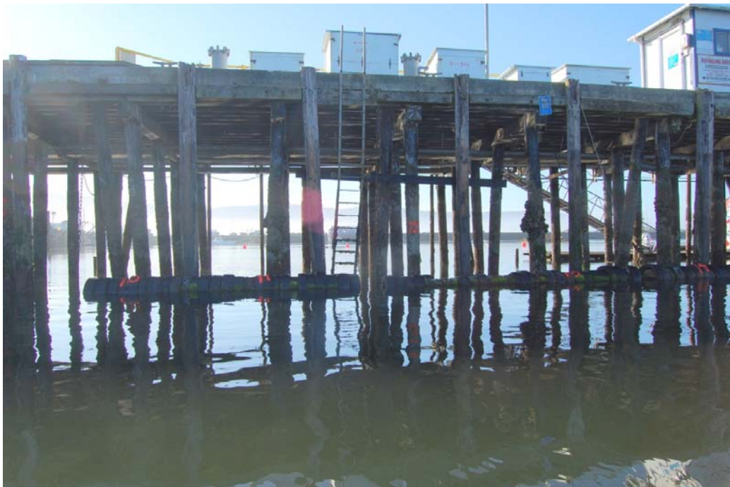
Approach Trestle Bents 10 to 13 (Photo #312) Steel ladder bent
