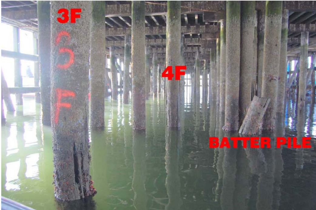
Piles 3F, 4F and batter pile (Photo #353)
