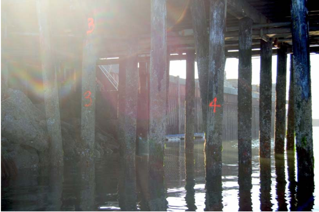
Approach Trestle Bents 3 to 4 (Photo #305) No damage noted
