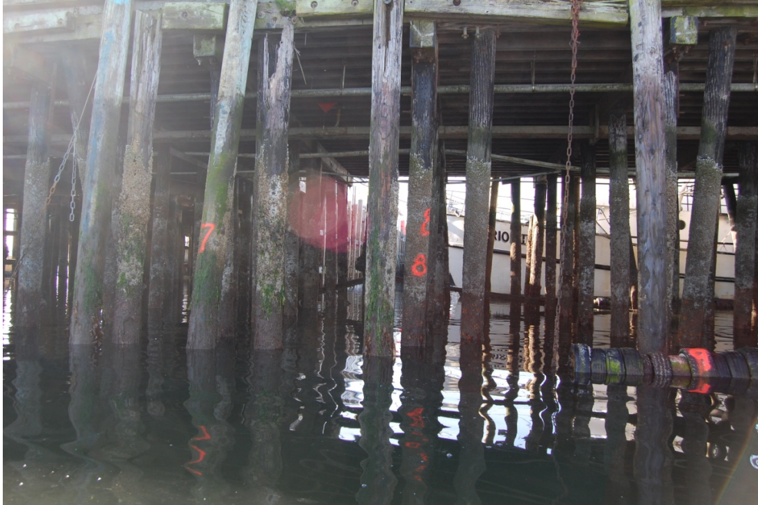
West Wharf Bents 6 to 9 (Photo #326) No damage noted
