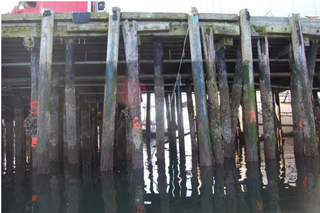
West Wharf Bents 5 to 8 (Photo #323) No damage noted
