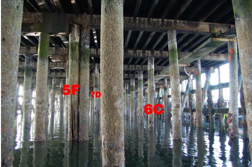
Piles 5F, 6C, and 7D (Photo #355)
