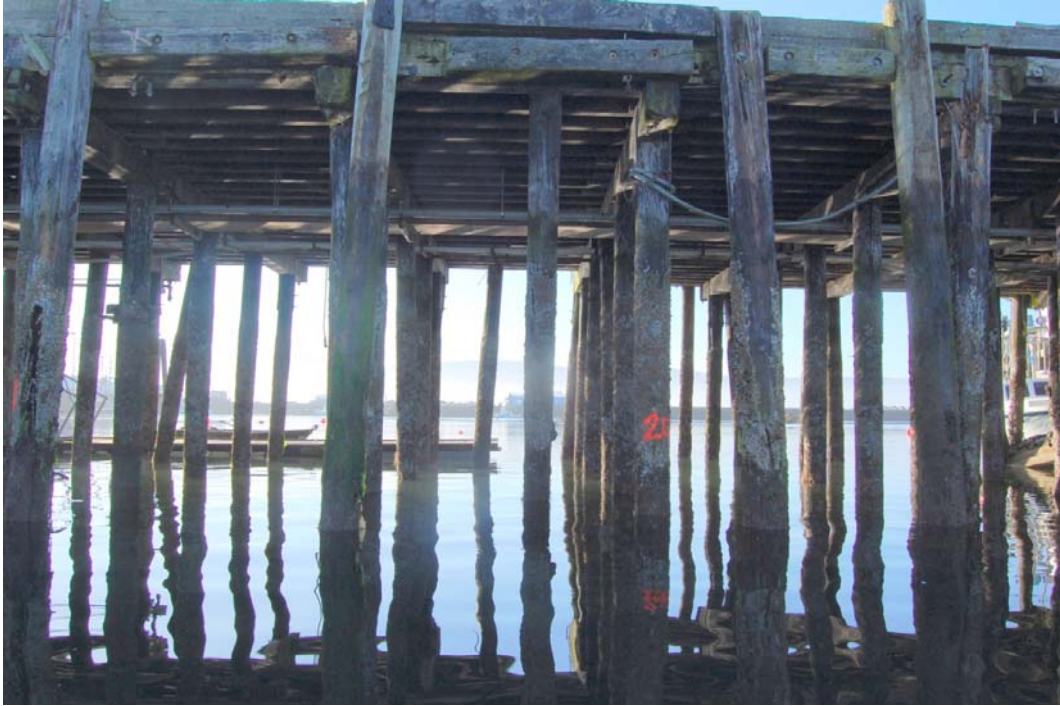
Approach Trestle Bents 19 to 20 (Photo #318) No damage noted
