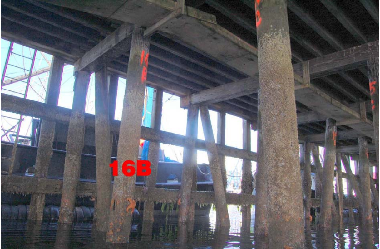
Pile 16B (Photo #362)
