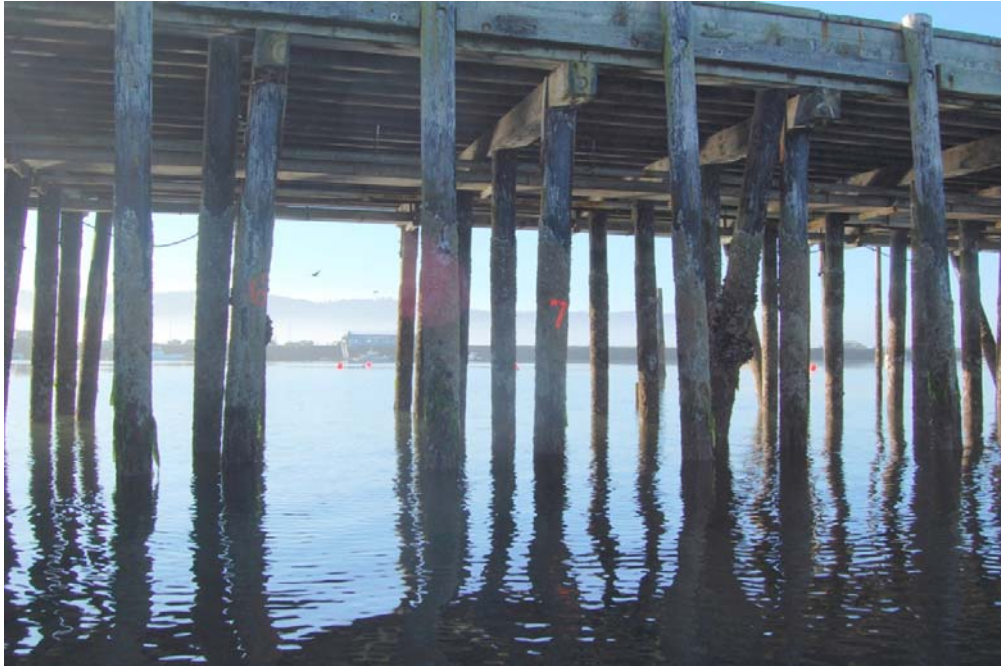
Approach Trestle Bents 6 to 8 (Photo #307) No damage noted
