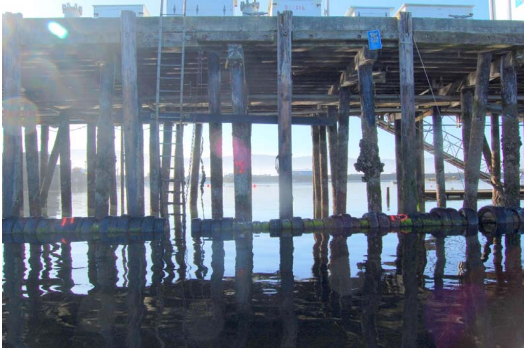
Approach Trestle Bents 11 to 13 (photo #313) Steel ladder bent
