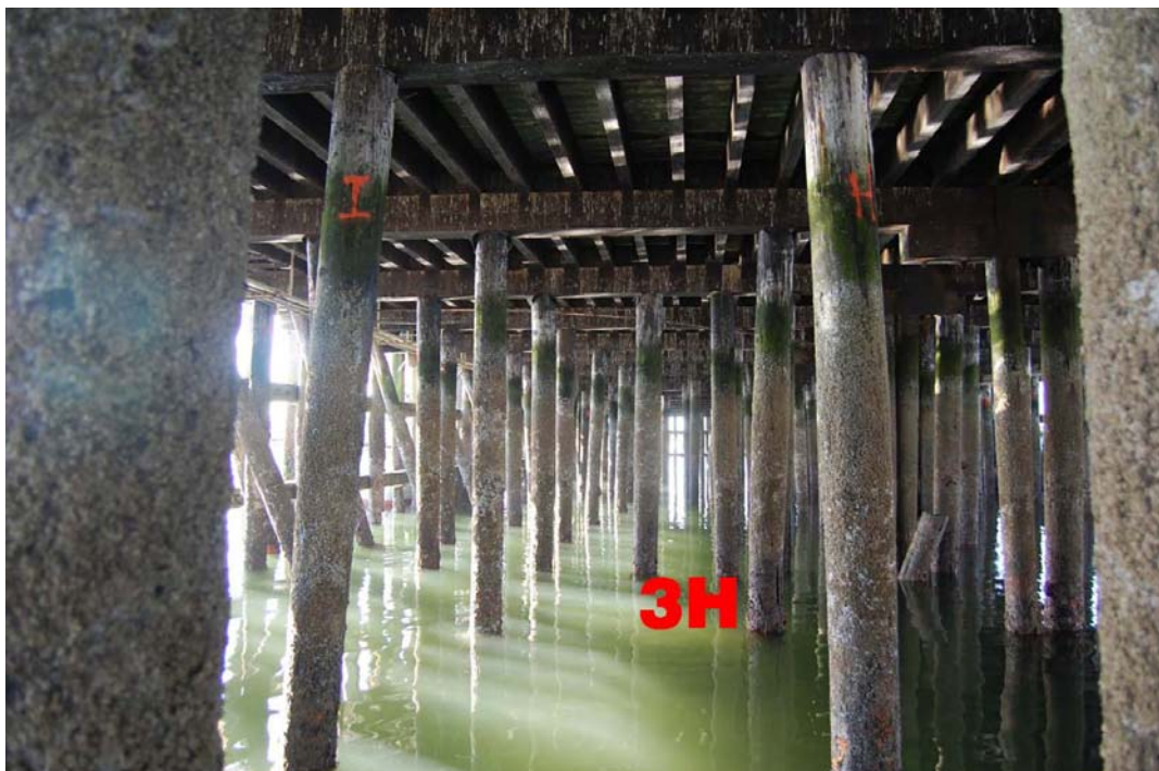
Pile 3H (Photo #348)
