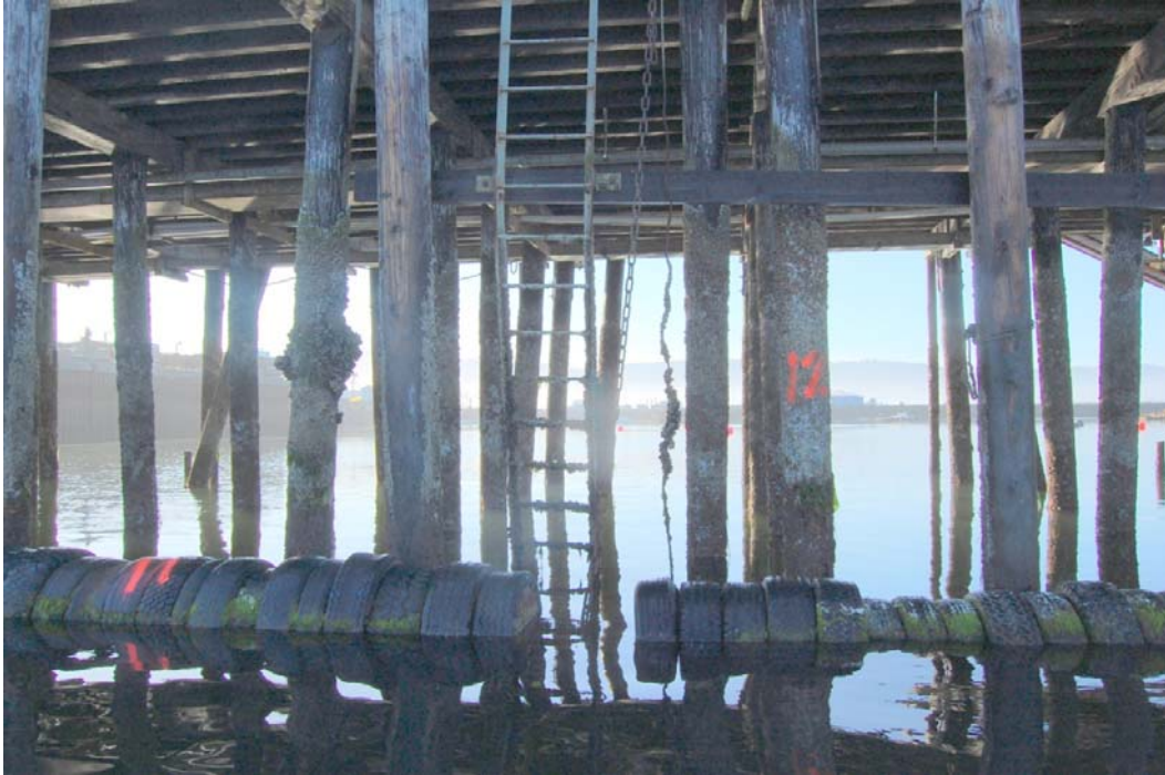
Approach Trestle Bents 11 to 12 (Photo #311) Steel ladder bent
