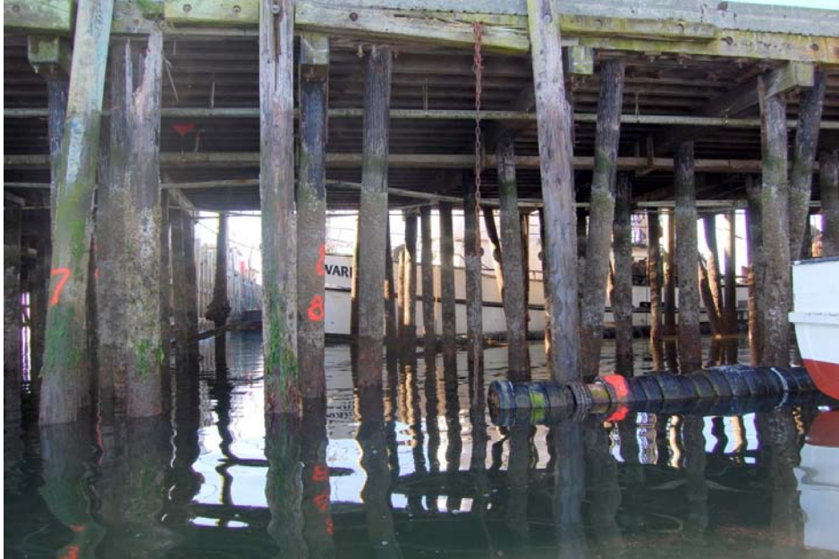
West Wharf Bents 7 to 10 (Photo #325) No damage noted
