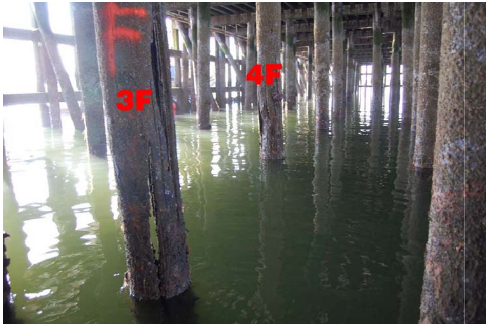
Pile 4F (Photo #354)
