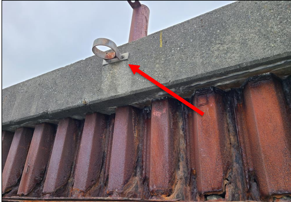
Photo 10. Typical Fender Pile Attachment Hardware
