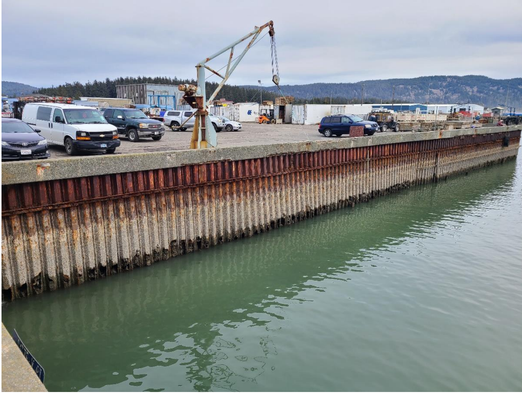
Photo 1. West-East Bulkhead, looking North
