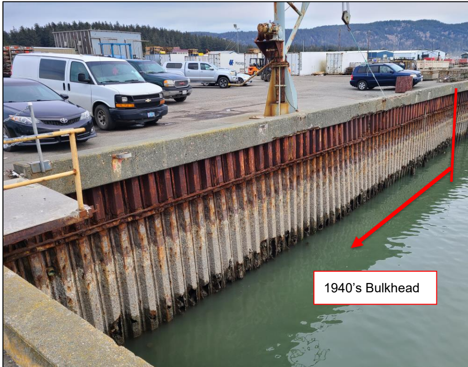
Photo 1. 1940's Bulkhead (STA 0+00 to 1+00)
