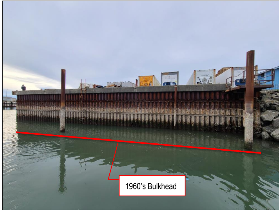
Photo 3. 1960's Bulkhead (STA 2+00 to 3+02)
