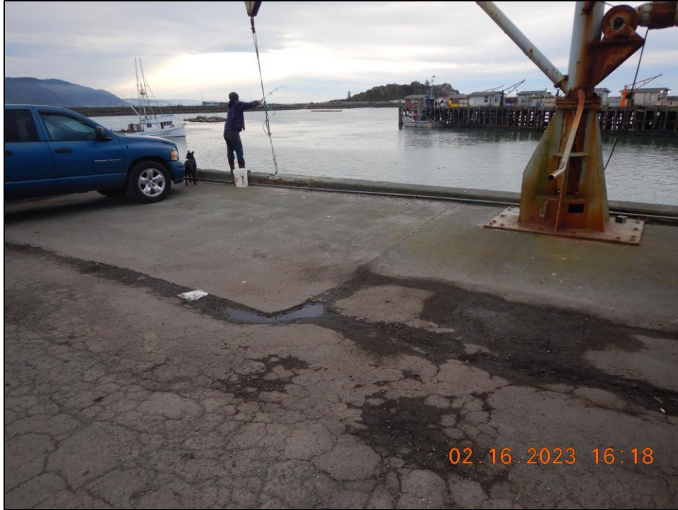
Photo 12. Concrete Pad Adjacent to the Bulkhead, Looking South
