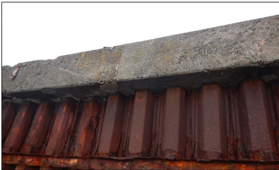
Photo 7. Typical Concrete cap, Looking from the Water
