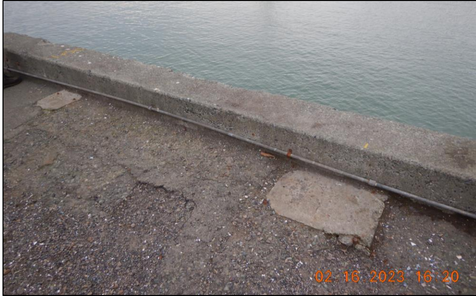
Photo 6. Typical Concrete Cap, Looking from the Yard
