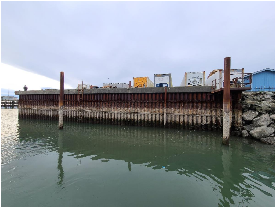
Photo 8. North-South bulkhead, looking west
