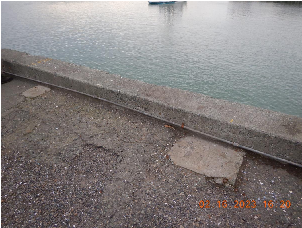
Photo 13. Typical concrete cap
