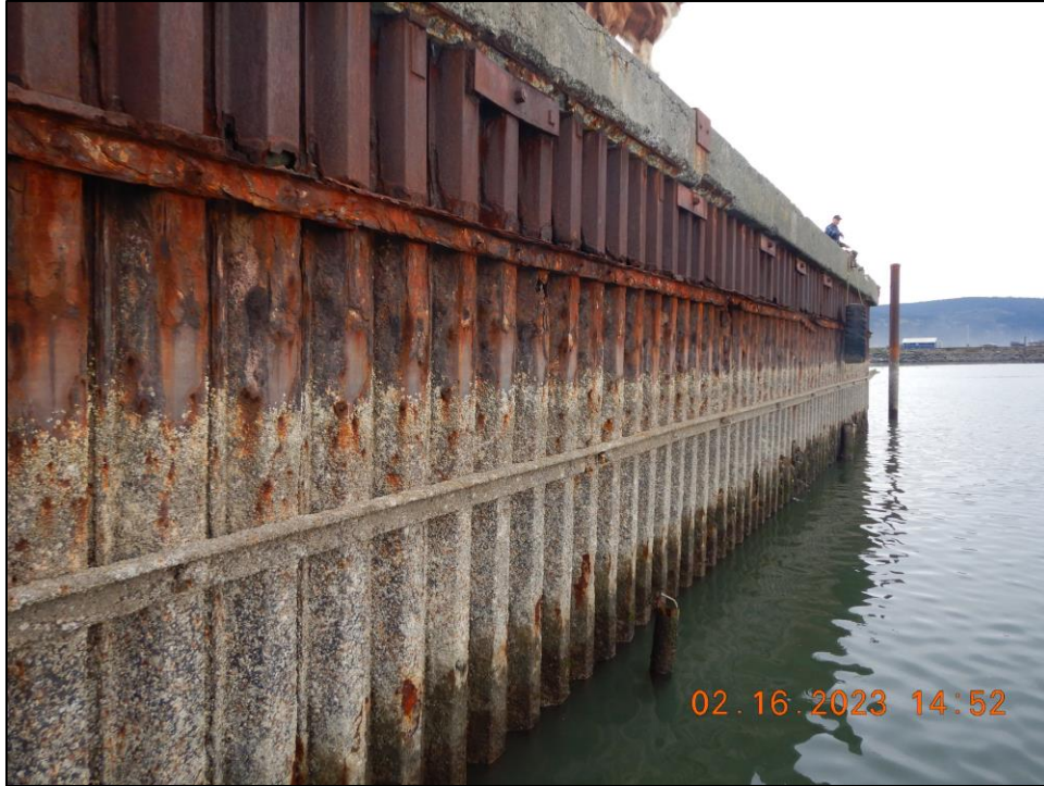
Photo 5. Typical Upper and Lower Waler from STA 1+00 to 3+02
