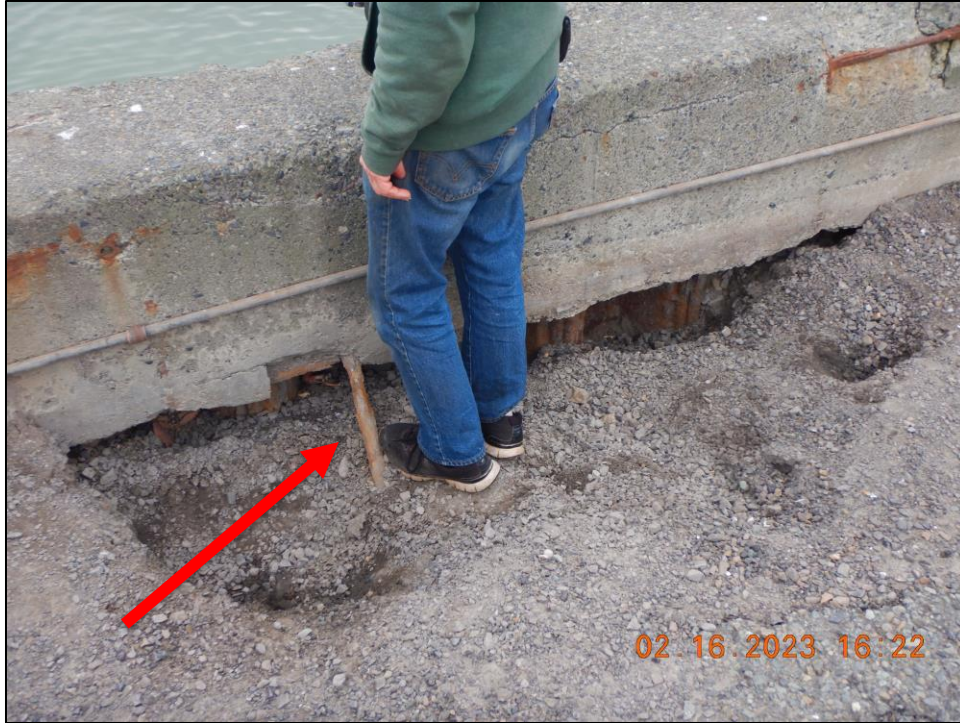
Photo 8. Angled Steel Tie Rod at Cap
