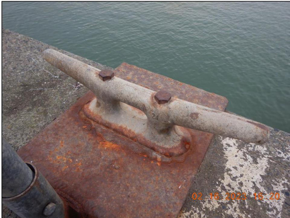
Photo 9. Typical 24-inch Mooring Cleat
