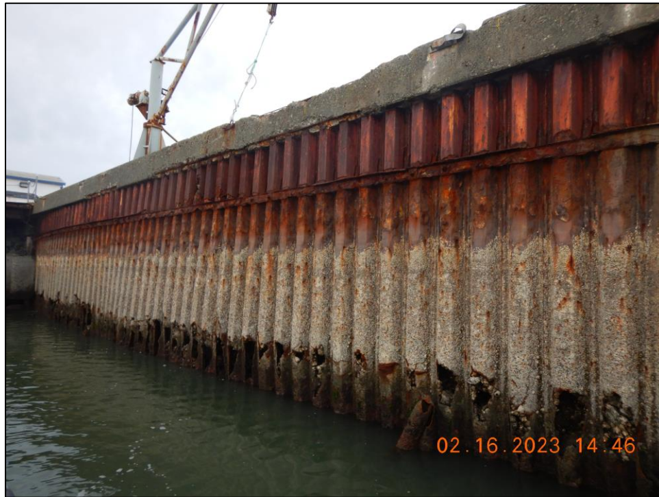
Photo 4. Typical Upper Waler from STA 0+00 to 1+00
