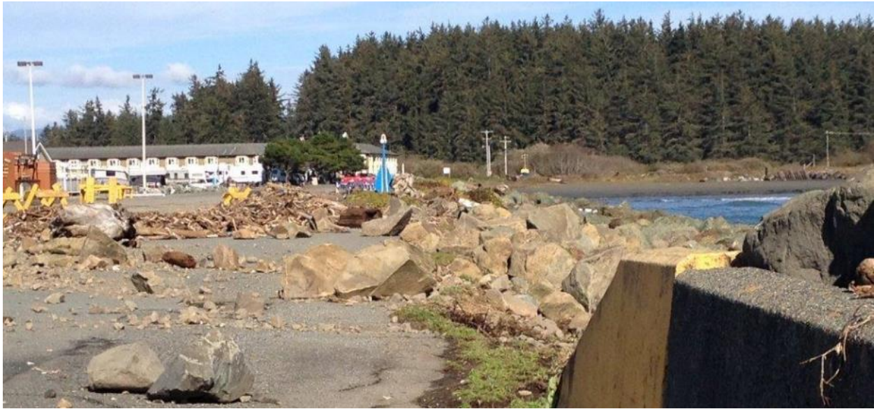
Image 1: Anchor Way Breakwater Debris from a 2018 Storm
