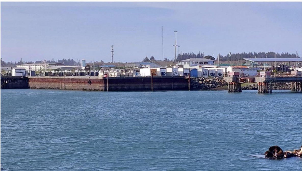
Long shot of entire Seawall (Figure 4)
